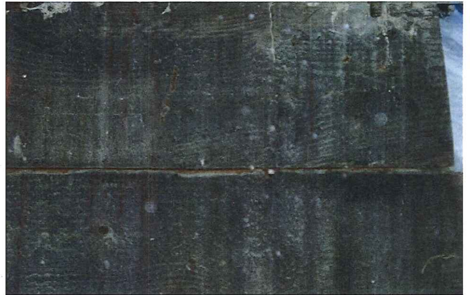
CK2199 Ballast Wall Timbers
